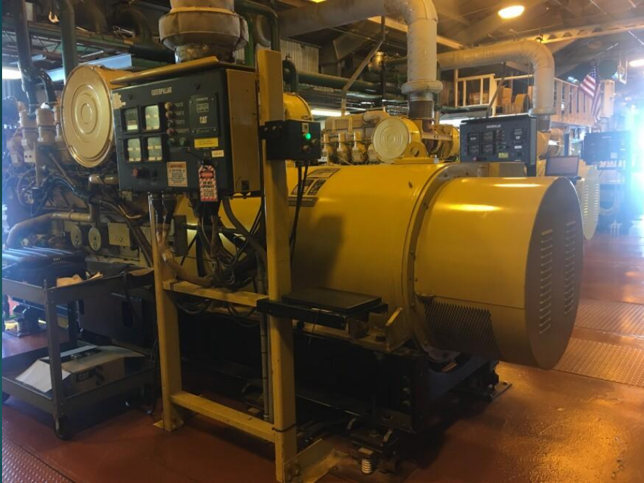
Diesel generator at Nushagak Electric's power plant in Dillingham, AK.
